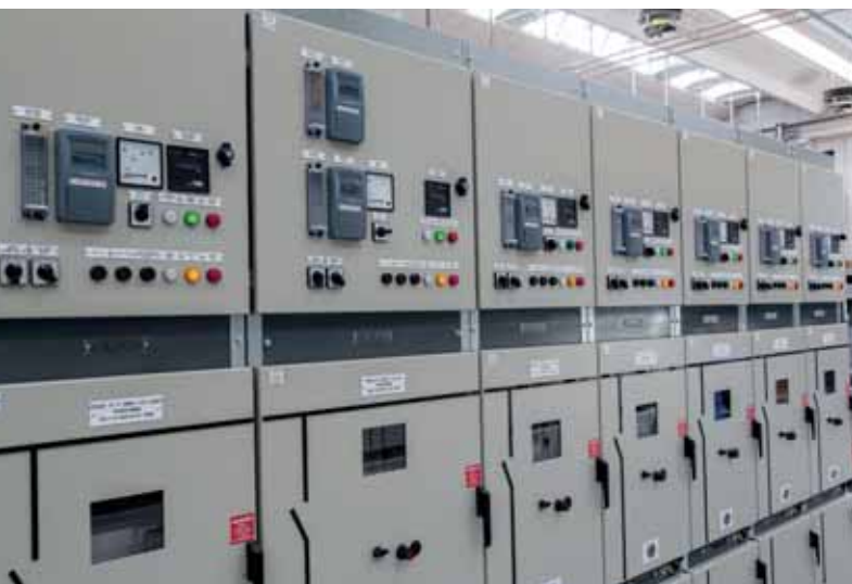
Quadri media tensione primaria Miniver C Miniver C primary medium voltage switchboards
