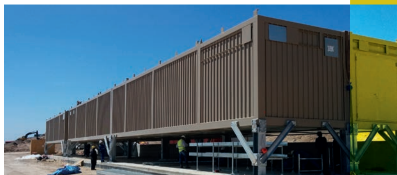
Cabine containerizzate Imesa Containerized Imesa's switchboards
