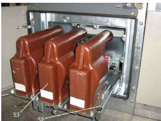
fig.55 – Voltage transformers removed from the VT compartment
