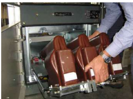
fig.51 – Placing/Removal of the voltage transformers
