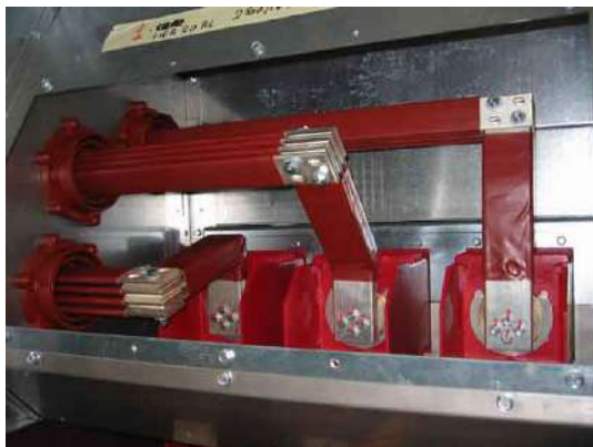
fig.20 – Distribution busbar compartment
