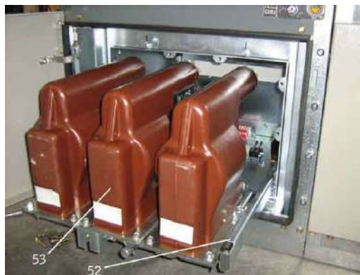
fig.18 – Voltage transformers on the withdrawable trolley
