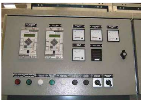
fig.19 – Low voltage compartment
