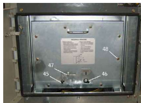
fig.54 – Voltage transformer compartment
