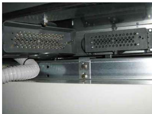
fig.46 – Connecting the auxiliary circuits
