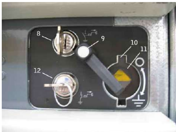
fig. 12 – Manoeuvring and key locking set of the earthing switch (unit front side)
