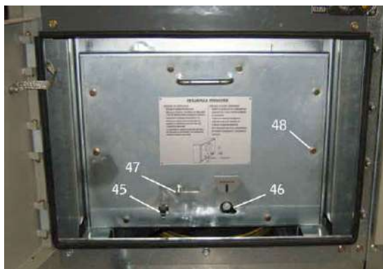
fig.17 – Voltage transformer compartment (front door open)
