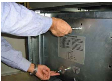
fig.53 – Placing/Removal of the voltage transformers
