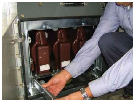
fig.52 – Placing/Removal of the additional guides for the VT trolley
