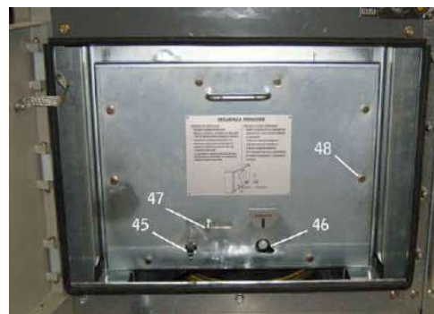
fig.54 – Voltage transformer compartment
