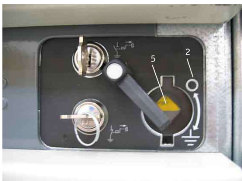
fig.10 – Manoeuvring and key locking set of the earthing switch (unit front side)
