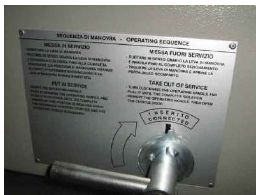
fig-57 – Putting in service / out of service the VT trolley
