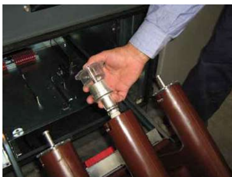
fig-59 – Replacement of voltage transformers fuses
