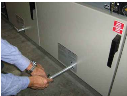
fig-56 – Putting in service / out of service the VT trolley
