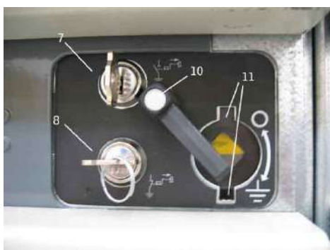
fig.58 – Manoeuvre seat for the earthing switch
